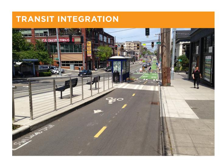
Bikeway design should consider locations of bus and other transit stops to reduce conflict both between bus and bike and with pedestrians accessing the transit stop. Signage and separating the bikeway from the transit stop support these goals.
