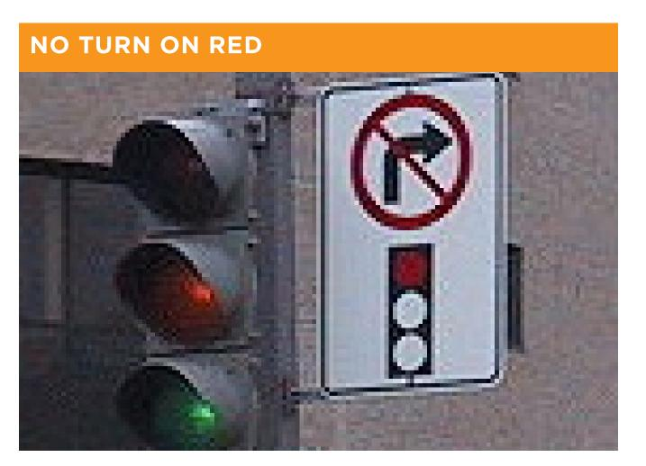
No turn on red restrictions prevent turns during the red signal to reduce motor vehicle conflicts with bicyclists and pedestrians. This restriction is commonly established at bicycle box installations, cycle tracks, and where bicycle signals are used to separate bicycle traffic from motor vehicles.
